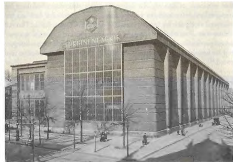
Figure 6: AEG Turbinenhalle, Berlin, Peter Behrens, 1909. The massive corner pillars show different tectonic features than the protruding, sleek glass curtain wall. Copyright: Siemens AG©
